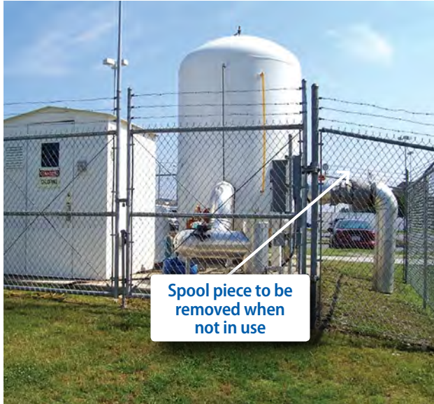
For accessible explanation of these two images about spool piece to be removed when not in use, and location of spool piece see Appendix G .
